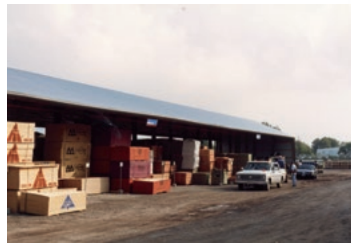
Stillwater's drive-through lumberyard
